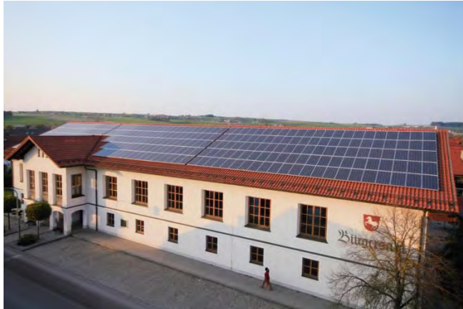
Figur 1 - Parallelmonterede solceller (Kilde: www.schletter.de )
